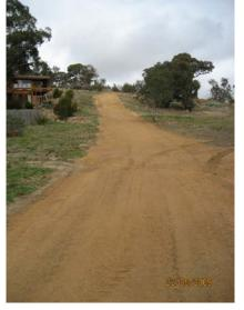
Paddy's River Granite was a convenient source of material for the job. Unfortunately, on steeper inclines, it was difficult to walk on without slipping. Much of the gravel eroded away (Photo 1) into the adjacent woodland.
